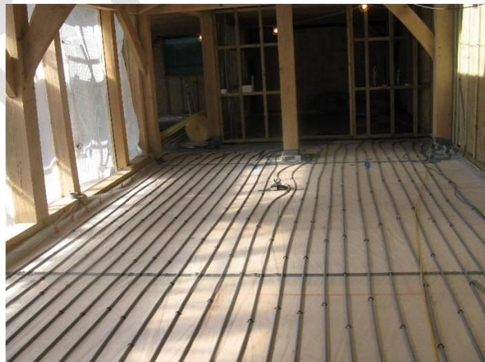
A typical underfloor heating installation consists of a circuit of pipe laid under the floor in a snake like fashion so that pipe is evenly spaced under the floor as shown in the photo above right (Oak house construction 10/4/2011)<sup>i</sup>.
